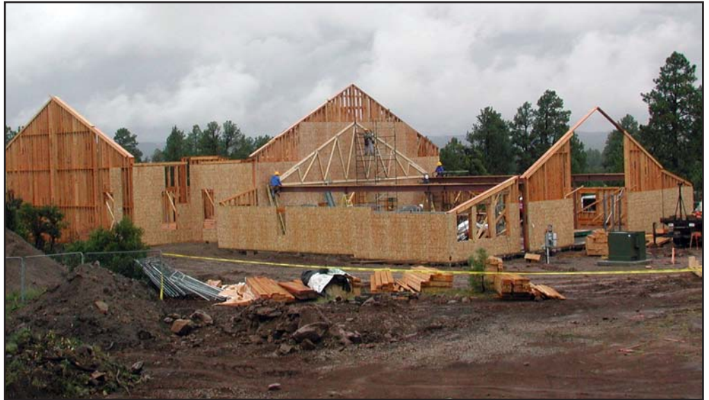
FCI works “rain or shine” for the roof to go up.
